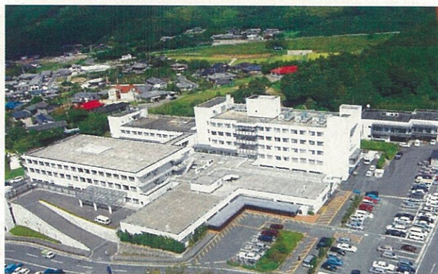
Hokusho Central Hospital
