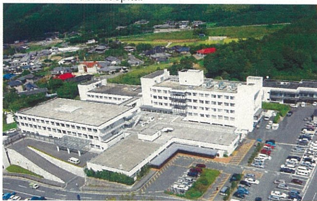
Hokusho Central Hospital
