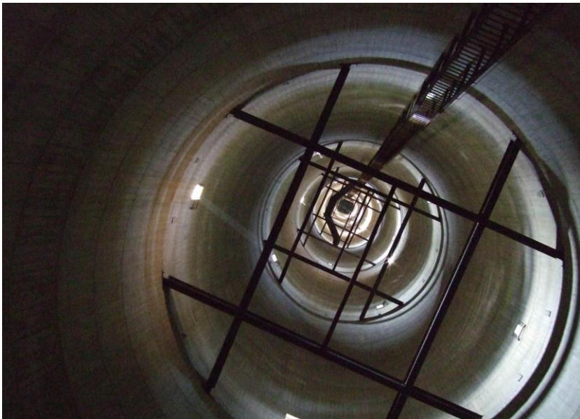
Fig.4 Inside of wireless tower
