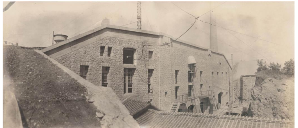
Fig.6 A picture of the transmission room under construction
